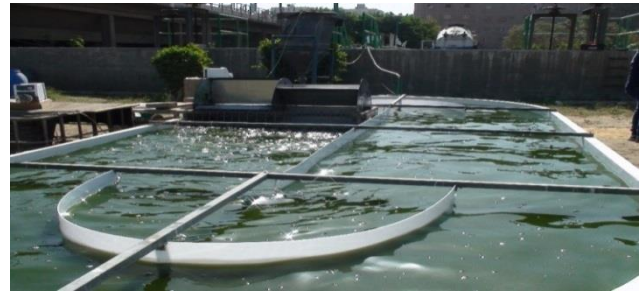
Figure 1. High rate algal pond system used for water treatment an algal biomass production
